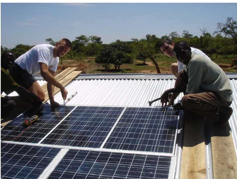
Assembly of the panels on the roof
