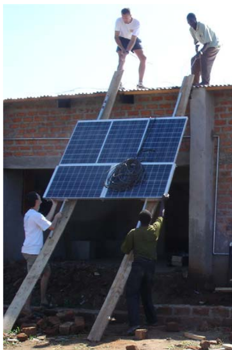
Panels are put on the roof
