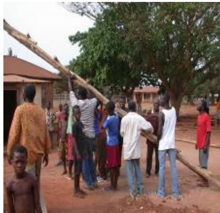
How to get to the roof...
