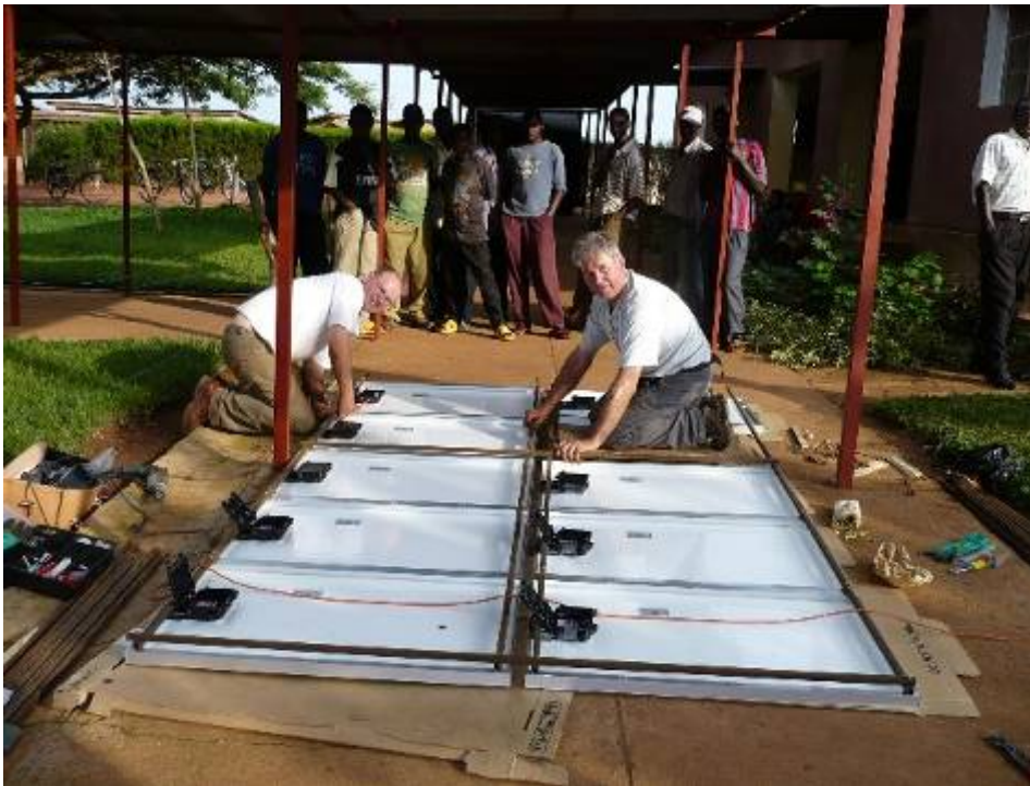
Johan and Axel assemble the PV panels
