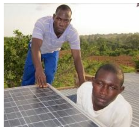
Practical works on the roof
