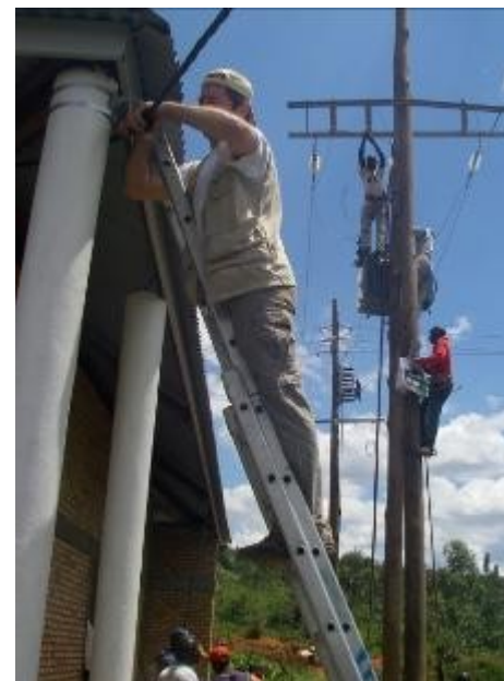
Jacques and local collaborators linking the transformer
