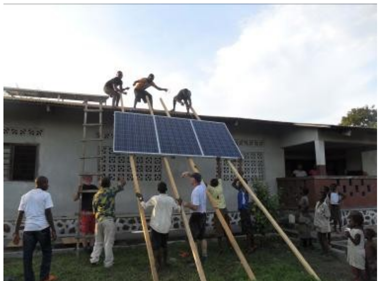
Set up of the panels-an always delicate operation
